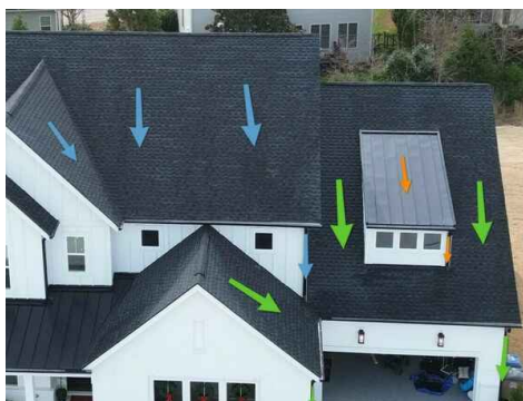
Flow to Garage Downspouts
